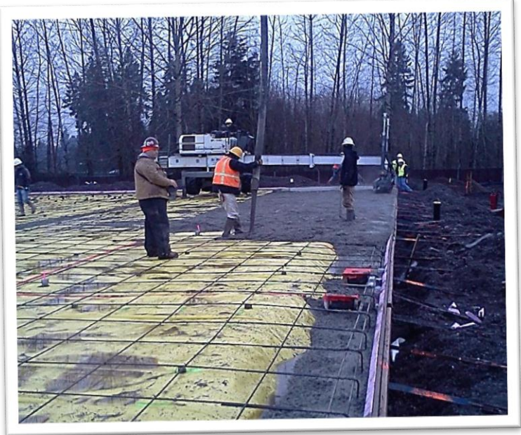
Columbia West testing rebar and concrete at the Goddard School.
