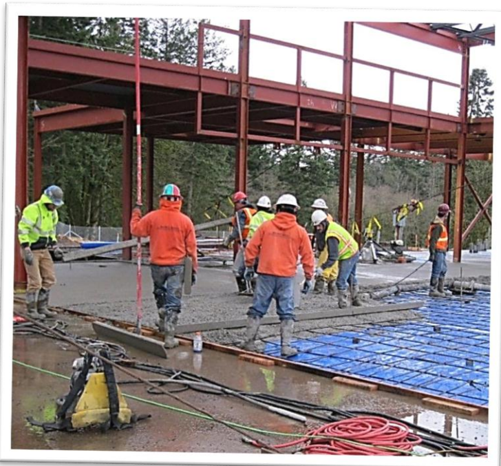
Columbia West conducting concrete testing at Woodburn Elementary School.
